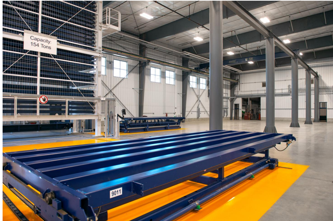
Premier Technology – Blackfoot, ID
